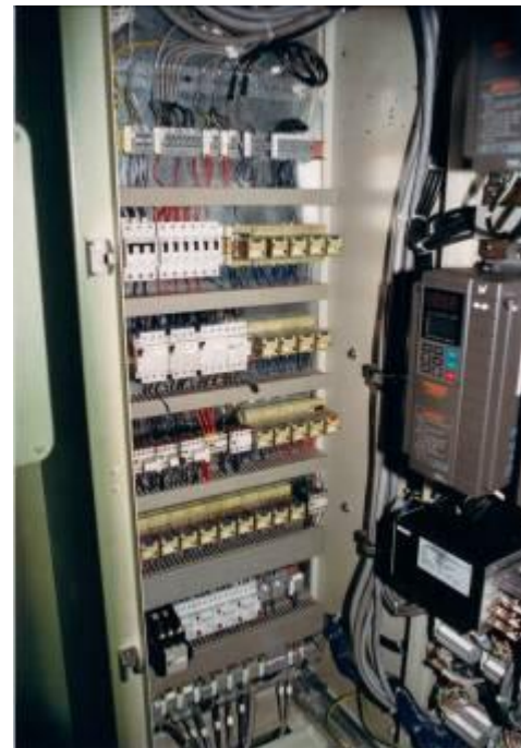
Figure 21: All the project the electrical part from the beginning was integrated.
