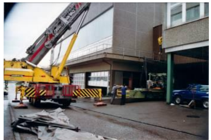
Figure 40: A sloping driveway with such a heavy machine requires great care and a good interaction between the people who carry out the transport.
