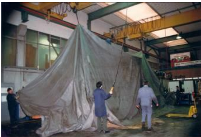
Picture 37a: lift this heavy Plan with the crane, was easier than by hand.
