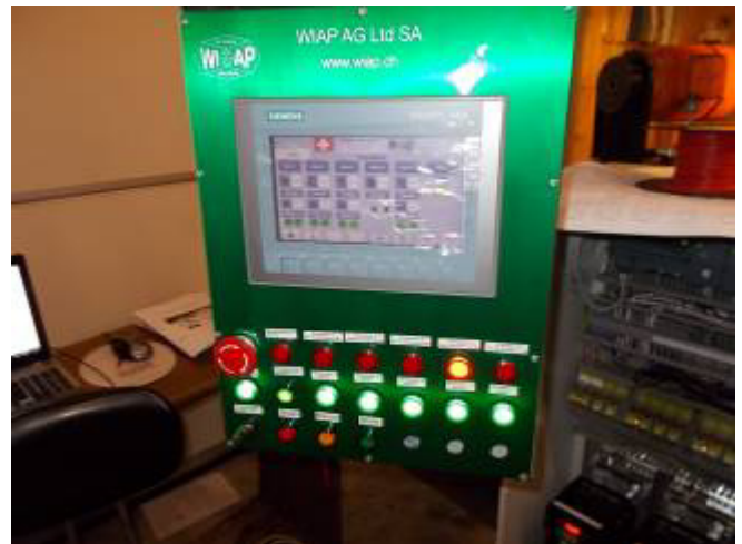
Das Panel in der Endmontage Phase. WU5130s
