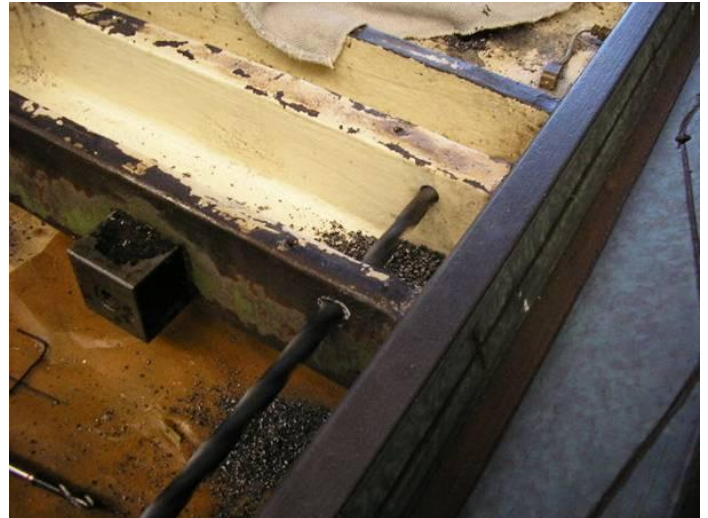
Figure 17: It takes a long drills and often the cast is quite hard, which is related to the cooling and the wall thickness of the respective zones, there must be drilled with tact WU_260_130
